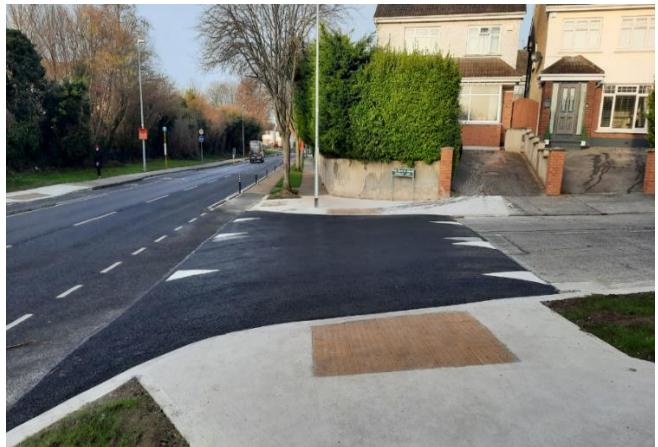
The provision of uncontrolled crossing locations give a safe defined crossing location along the route. These crossing points include tactile paving and drop kerbs which allow a safe crossing location for all road users.
