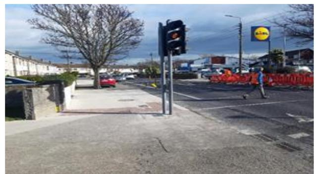
Upgrade of Tactile Pavement and Surrounding Footpath – Grange Road (Signal heads to be replaced later to ELV type)
