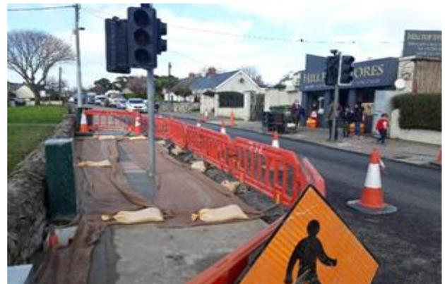
Upgrade of Tactile Pavement and Surrounding Footpath by The Hill - Malahide, (Signal heads to be replaced later to ELV type)
