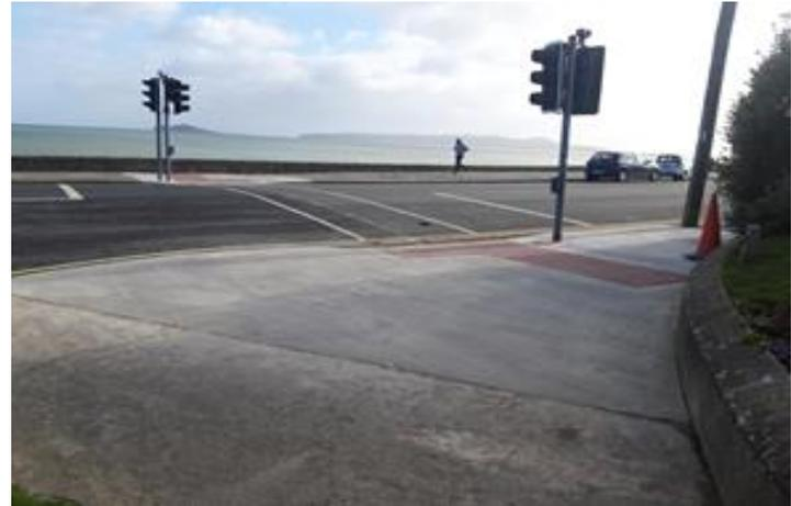
Upgrade of Tactile Pavement and Surrounding Footpath by Wendell Avenue-Coast Road, (Signal heads to be replaced later to ELV type)
