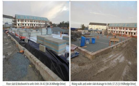
Floor slab & blockwork to units 34-42 (18-26 Kilhedge Drive)
