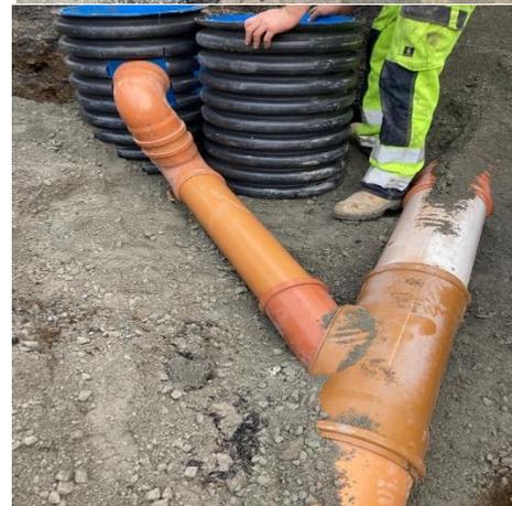
A 140m long storm water pipeline and road gullies was installed on St Margaret's Rd, Avenue, and Church Rd Malahide to relieve flooding on St Margaret's Rd and New Street Malahide. The existing road gullies were separated from the foul sewer in the area which will reduce the volume of water entering the foul network during storm events.
