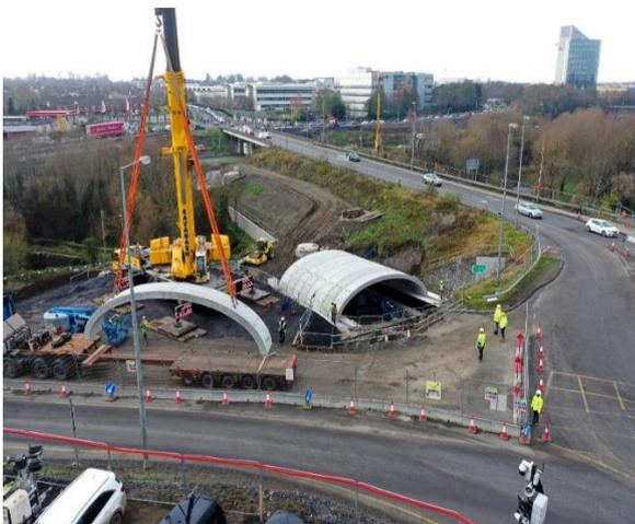
Major bridge construction works were undertaken in December where an arched underpass was installed over the course of two days. Piling works for bridge abutments has been completed this month and retaining walls on adjacent roads are currently being built. Piling works for the central pier will be concluded in January with significant traffic management to be put in place on the N3 from January onwards to facilitate these works.
