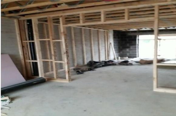
**Stud walling and ceiling joists at house in Hyde Court Rush**
