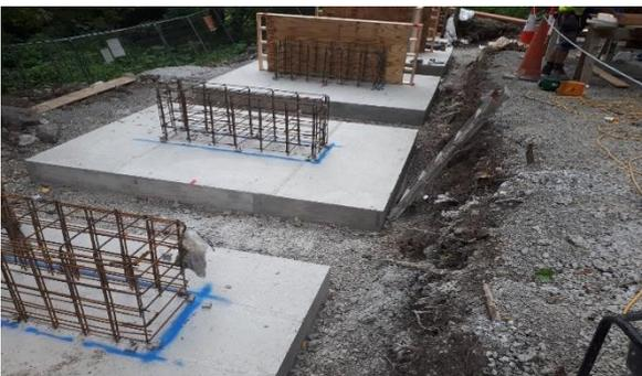
**Steel fixing and installing formwork to columns and abutment walls**
