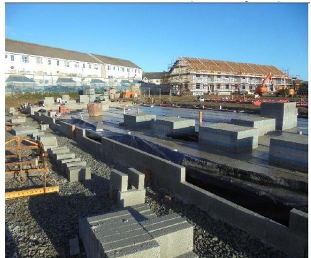
Floor slab & blockwork to units 43-51 (27-35 Killhedge Drive)
