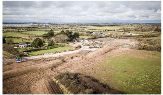
The main activities currently taking place on site include setting out of the alignment and earthworks, excavation for road sub-structures and construction of the road drainage network. One of the most visible elements of the contract will be the earthworks phase and this will take place in the coming months when ground conditions are more favourable.
