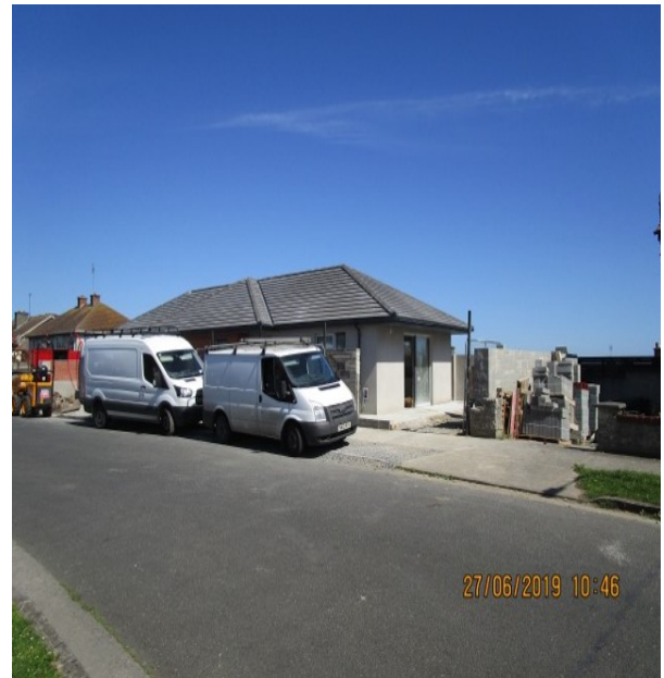
Pinewood Community Refurbishment - 2 houses
