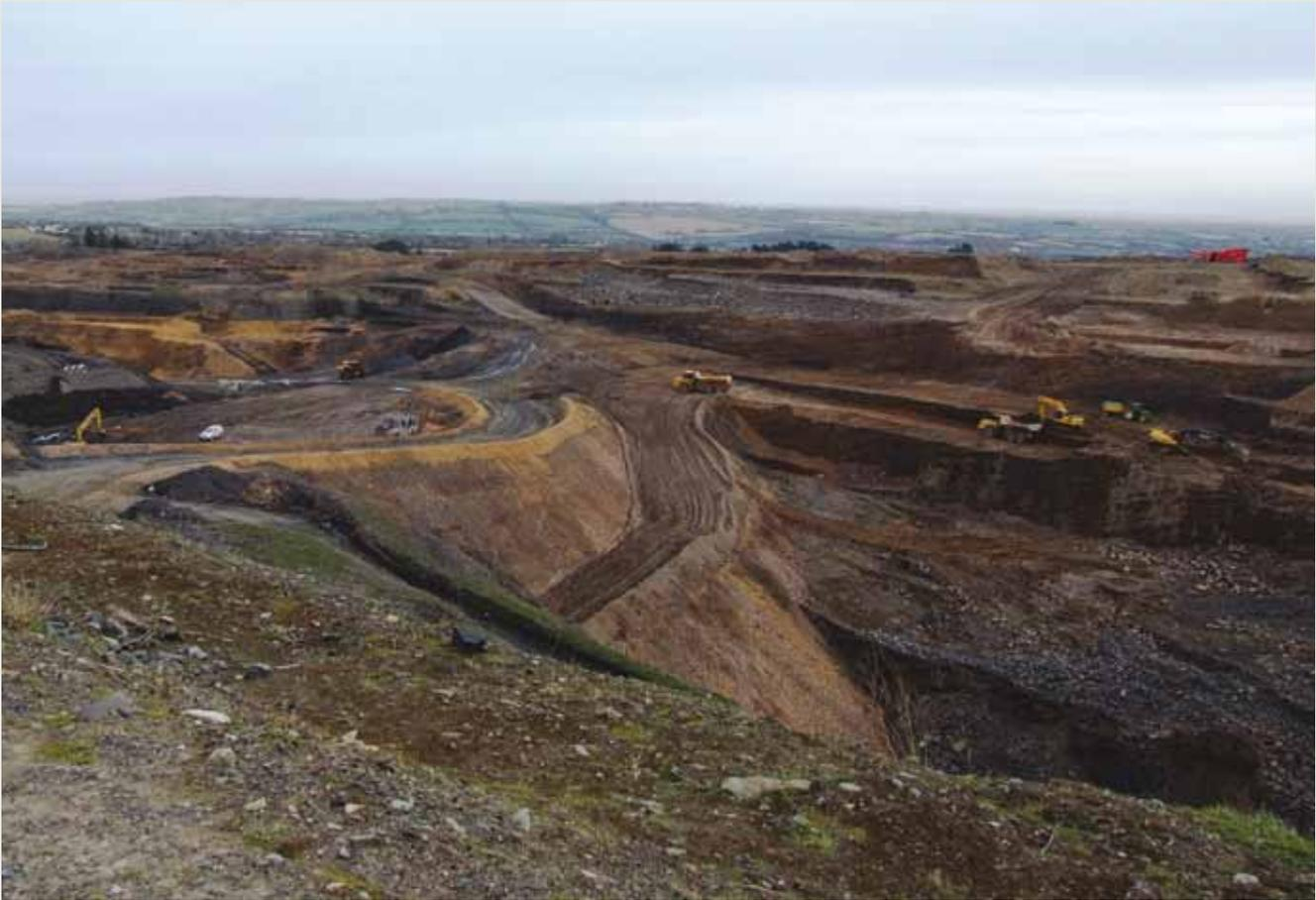
A view northeast into Nags Head Quarry, which will eventually be filled with waste in environmentally engineered cells
