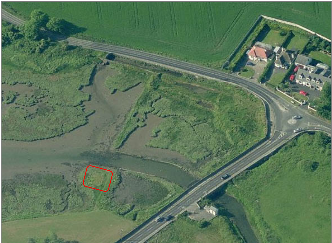
11. Oblique aerial view of mill from north ( www.bing.com/maps ). The foundations of the mill building are indicated by the red rectangle.
