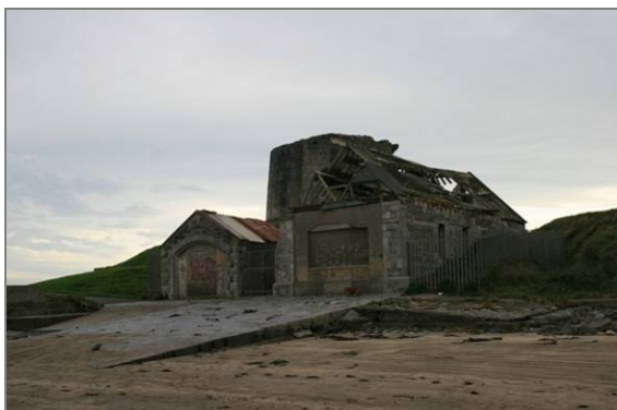
18. Former Balbriggan lifeboat station
