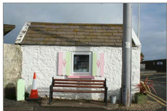
17. Former life boat boathouse, Skerries Pier. (Site No. 11, Appendix 3)
