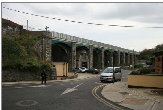
19. Balbriggan viaduct with RNLI boathouse
