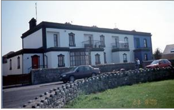
24. 20 th Century former lighthouse keepers' houses, Skerries: built for keepers of Rockabill Lighthouse.
