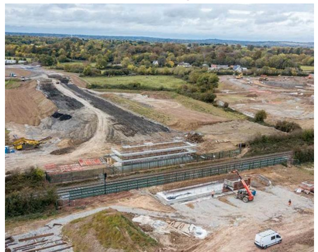
Road Widening Near Donabate Railway Bridge (R126)
