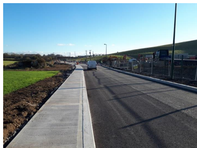
Balleally Landfill SW Scheme Construction Works October 2018
