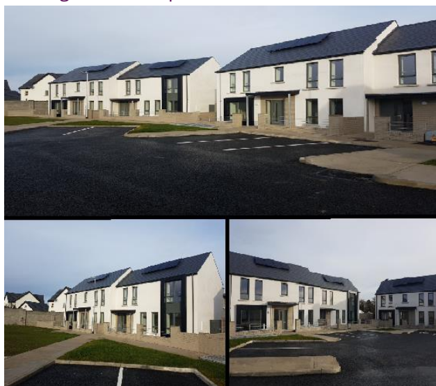
New social housing nearing completion at The Grange, Ballyboghil
