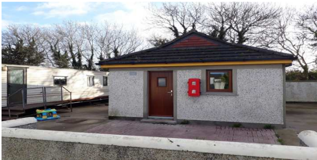
New fire safety installations at St Macullins Park
