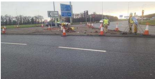
Works Ongoing - Dublin Airport Roundabout
