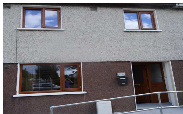
Example of Window & Door Replacement in Dublin 15
