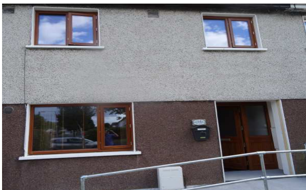
Example of Window & Door Replacement in Dublin 15
