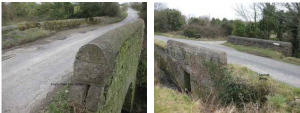
Knightstown Road Bridge Colecott Bridge
