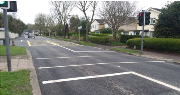
Roadworks at Swords Road/Millview Road junction are now completed:
